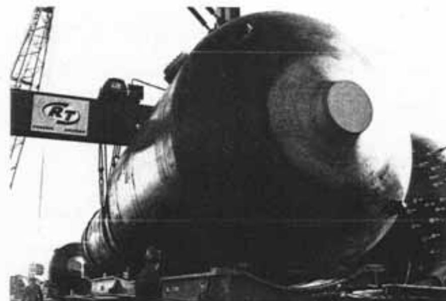
340 ton steam generator is lifted clear of rail cars.
